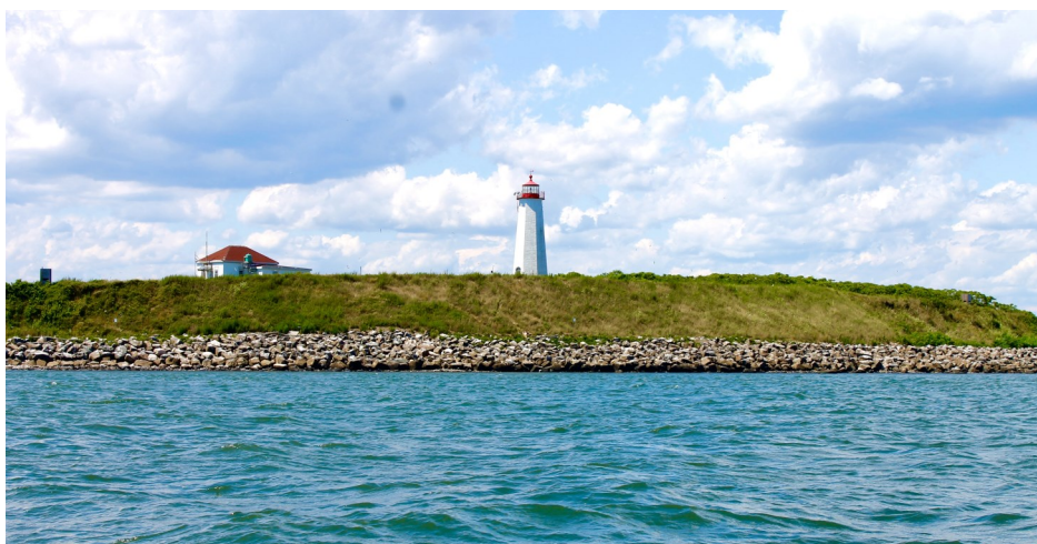
The back or eastern side of Faulkner's Island illustrates Phase 1 of the traprock (igneous basalt) stone revetment protecting the lower embankment for approximately 1000 linear feet. The upper embankment has been reduced in pitch with a hardy cover of vegetation.
