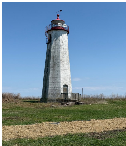
Faulkner's Lighthouse with weed mat and mulch in the foreground. Island is prepped for the return of the terns.
